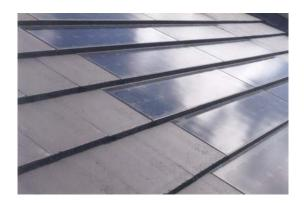
Solar panels integrated within the roof
