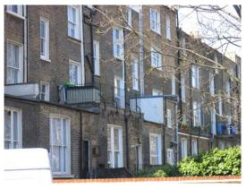
A relatively unaltered rear elevation of a terrace built with a shallow full width rear extension up to ground floor – any alteration would undermine the original unity
