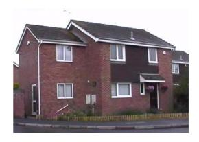
The ridgeline of this side extension is lower than the main house but the eaves line remains at same level.
