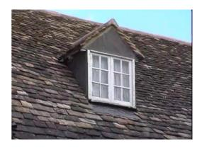
A traditional pitched roof dormer located well below the ridge of the roof.
