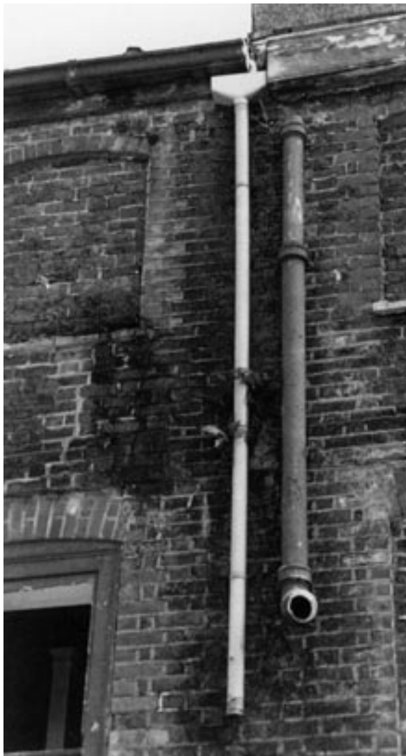
Defective gutters and pipes have caused severe damage to this listed house. (Wandsworth)
