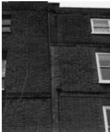
Structural cracking from long term movement can still be repaired
