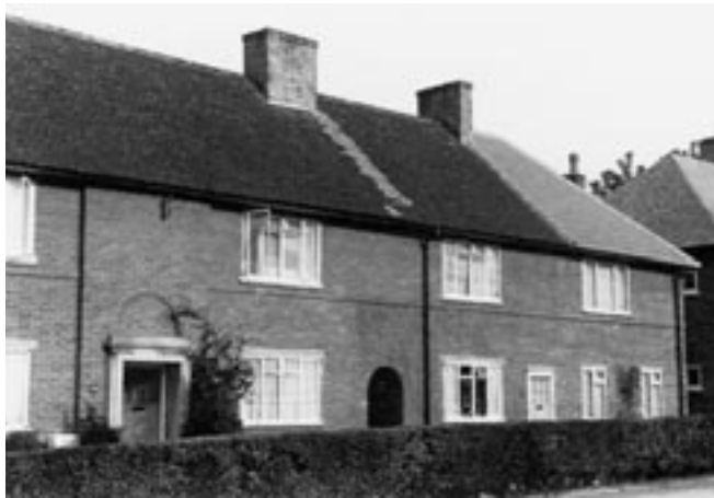
Contrasting roof material and obvious join spoils the group (Roehampton)
