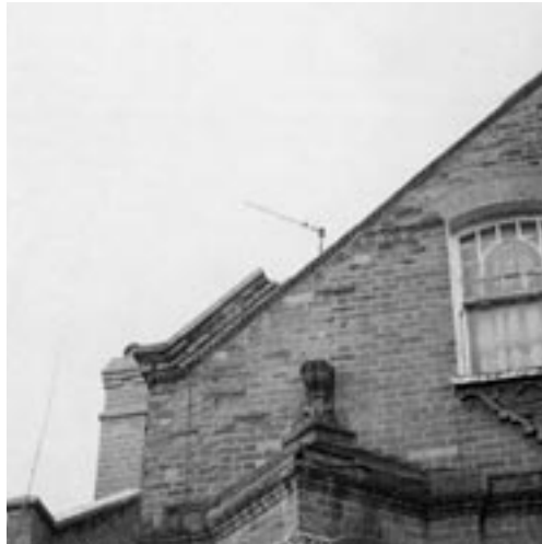
Poor brick repair and loss of the rich cornice have disfigured this house. (Tooting)
