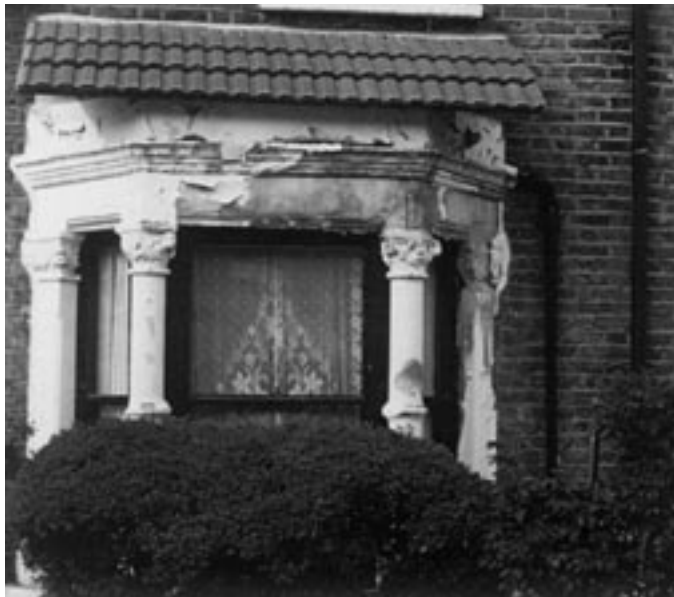
Dampness – leading to decay, rot and failure of materials
