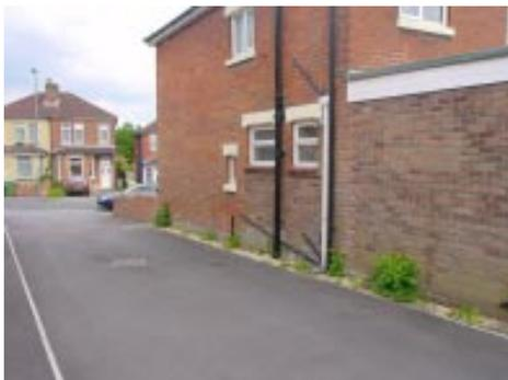
*These plastic service pipes look unsightly and can easily be damaged on this access road*
