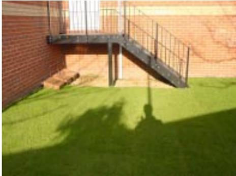
*The space below this staircase should have been finished with paving and the gas meter boxes cannot be easily accessed in this location*
