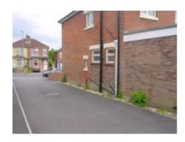
These plastic service pipes look unslightly and can easily be damaged on this access road
