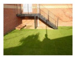
The space below this staircase should have been finished with paving and the gas meter boxes cannot be easily accessed in this location
