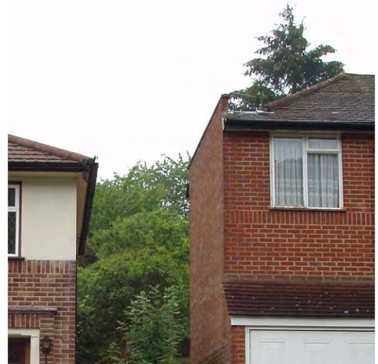
*Fig 30 - An example of a parapet built to avoid an eaves and gutter overhang. This should be avoided.*
