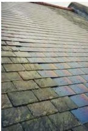
Figure 10 - Photovoltaic roof tiles compared to regular roof tiles
