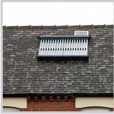
Figure 9 - Solar water heating panels.
