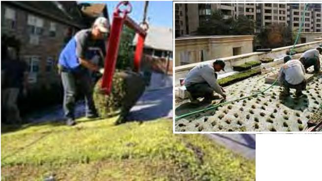
Figure 17 - The laying of an extensive green roof. Sedum Blankets rolled on top of a felt roof.
