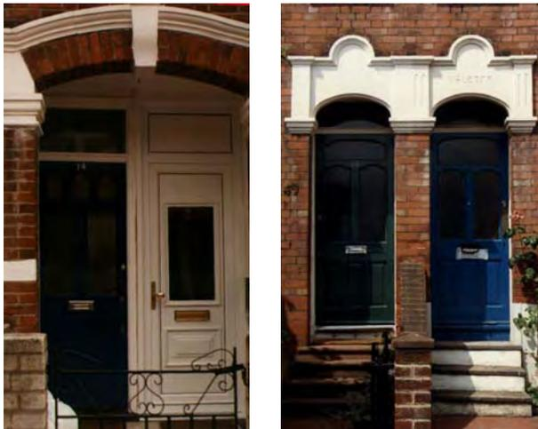
*Fig 34 - The replacement U.PVC white door fails to reflect the architectural details of the house. The photograph on the right shows original Edwardian front doors.*
