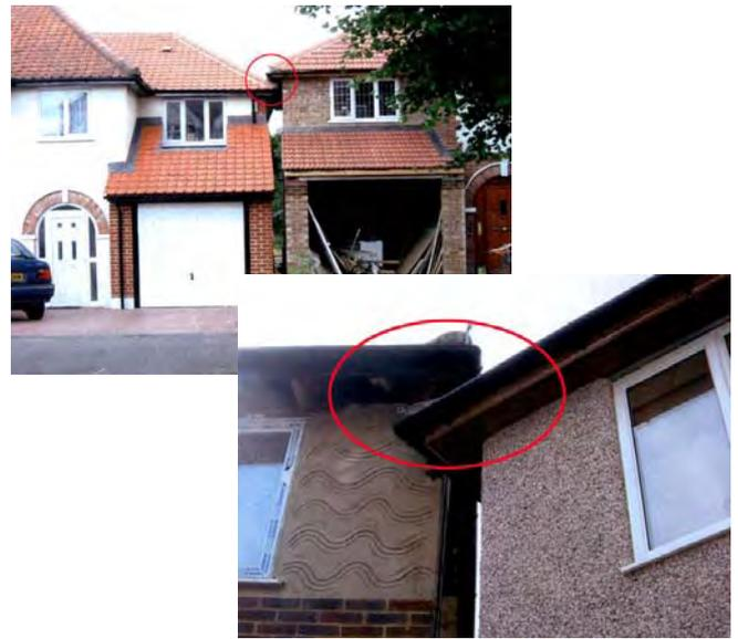
*Fig 6 - Examples of extensions which have not made allowances for eaves and gutter overhang*
