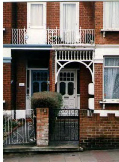
*Fig 35 - Removing decorative timber trellis from the house on the left has upset the balance of this pair of doorways*
