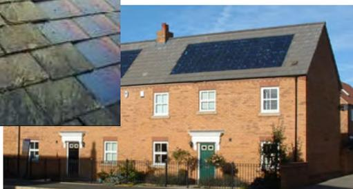
Fig11– Photovoltaic panels on a terraced house
