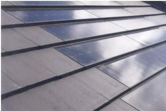
Solar panels integrated within the roof
