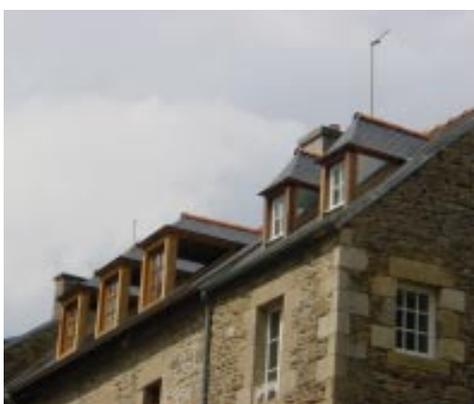
*Dormer windows in Brittany, France, use a simple construction allowing the sides to be glazed*
