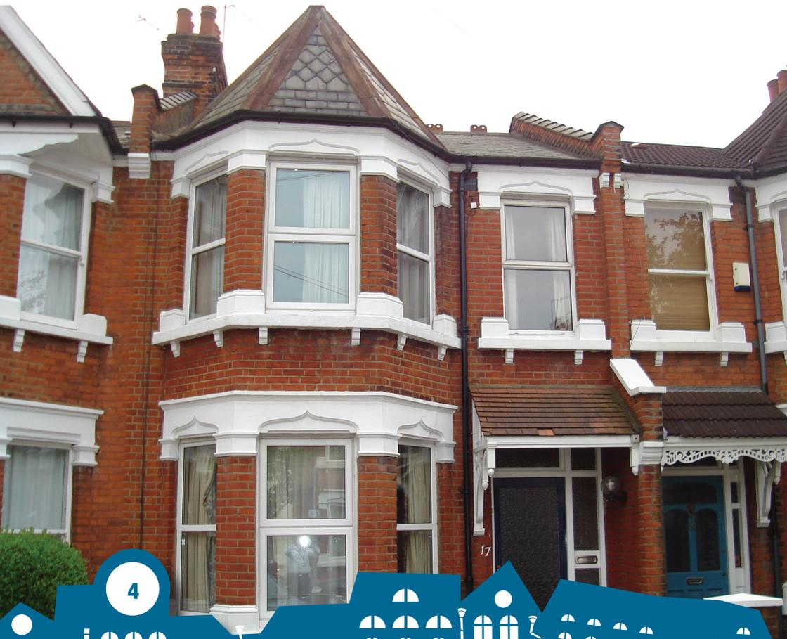
Many houses in the SPD area have 2 storey bay windows with pitched roofs with a pointed gable facing into the street. Generally the bay should be extended to the additional floor, with the bay window roof replicated at the new level, as shown in Figure 4 and Figure 5 below.
