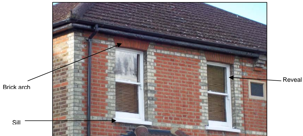
Diagram 9: Components of a window and opening
