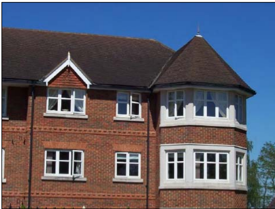
Roof, brick and stone detailing
