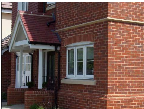
Brick and stone detailing
