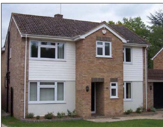
Balanced front extension to a detached property
