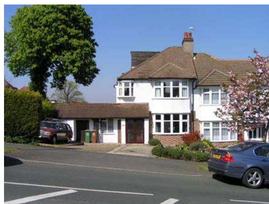
Figure 17: Too wide and the side extension detracts from the dwelling and streetscene.
