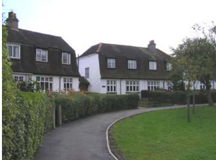
Figure 16: Individually these buildings would not be listed, but as a group they create a pleasing streetscene in a Conservation Area.
