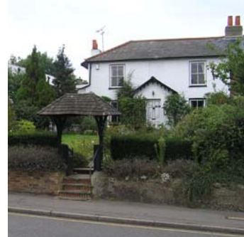
Figure 15: A Grade II Georgian listed building in Sutton.
