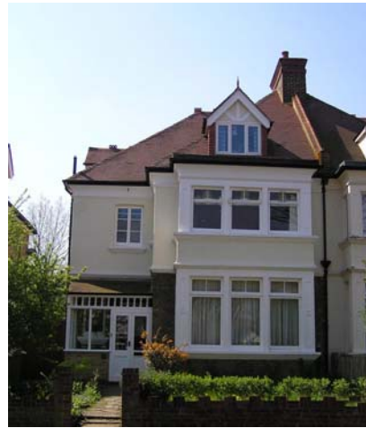
Figure 26: The Edwardian dormers are 'original' and sit comfortably within the roofscape
