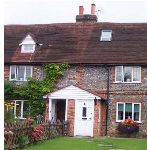
Figure 23: Poor quality porches hide traditional details.
